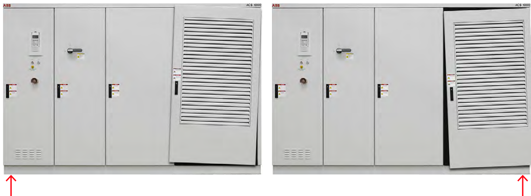
Figure 6-1: Leveling the drive
